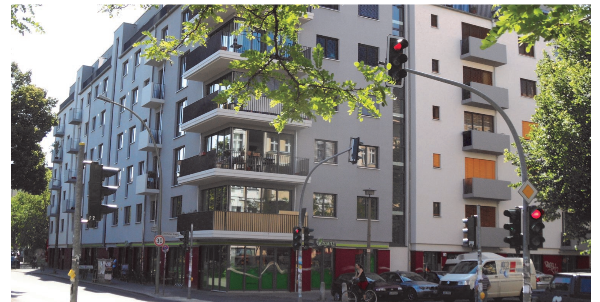
Photo 1: Multi-storey passive house at Arnimplatz, Berlin-Prenzlauer Berg built for 123 persons (41 dwellings) and covering an area of 4,600 m 2 .
